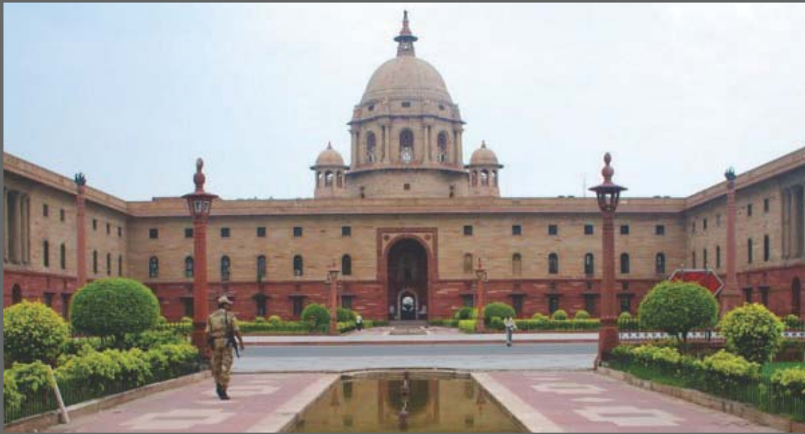
Rashtrapati Bhavan, Delhi | Waterproofing by IWL
