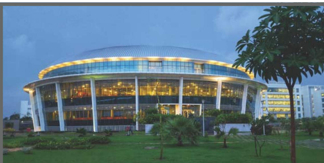
HCL Sholinganallur, Chennai | Waterproofing by IWL
