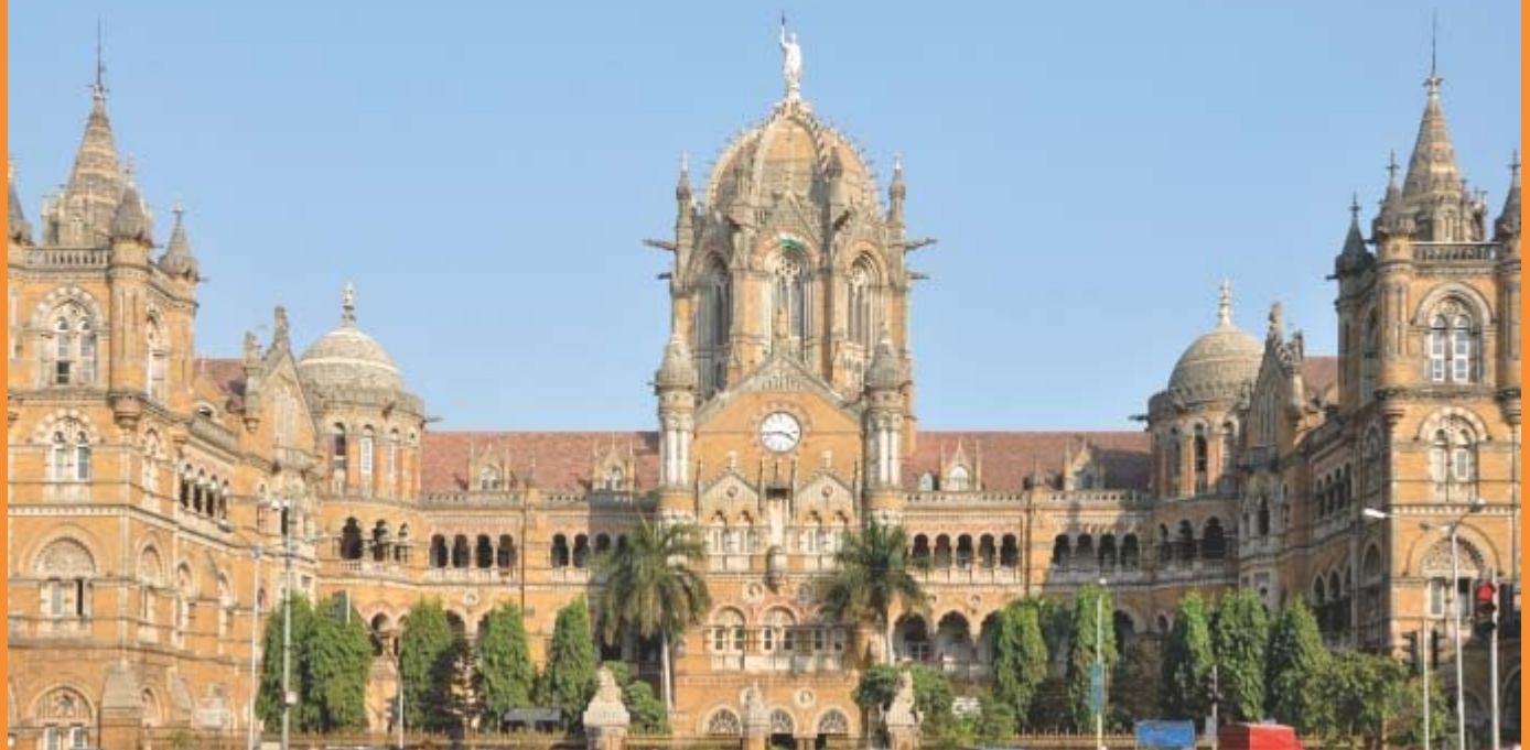
Chhatrapati Shivaji Terminus, Mumbai Waterproofing by IWL
