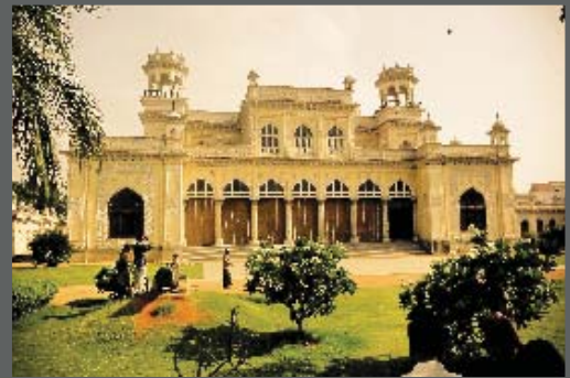
Chowmahala Palace, Hyderabad Waterproofing by IWL
